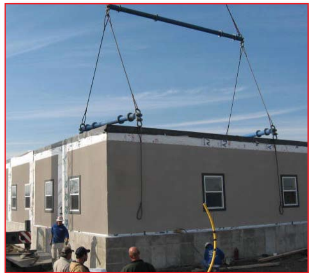
A crane sets the final module in the clinic’s construction.
