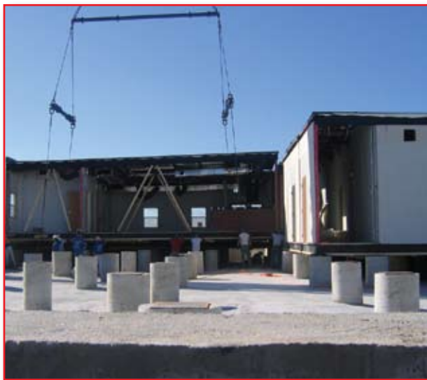
Each module is carefully fitted to adjoining modules.
